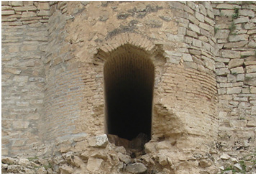
Fig. 6: Outlet of gallery number 3 and the application of bricks and rocks in Saroj mortar
