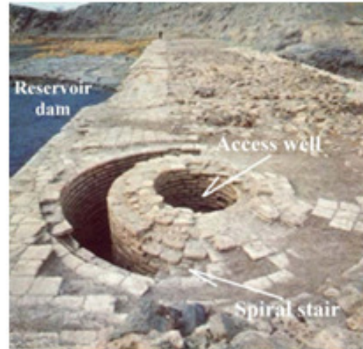
Fig. 2: brick well and the stair case of Golestan dam for accessing the intake valves
