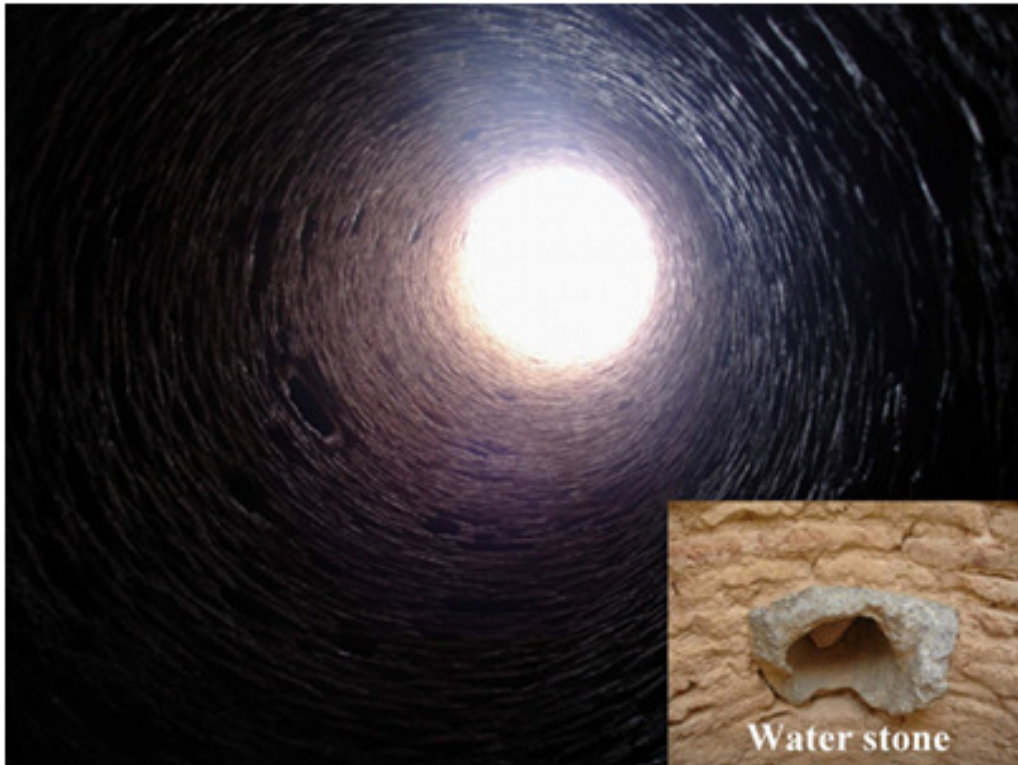
Fig. 7: vertical well of the spillway number 2 and the water stones used for water withdrawal
