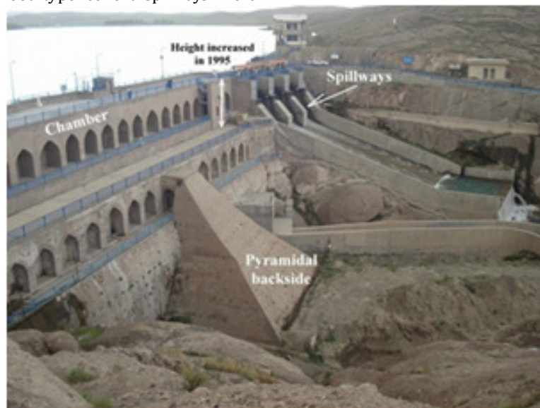
Fig. 3: Fariman dam after reconstruction and increasing the height in 1995
