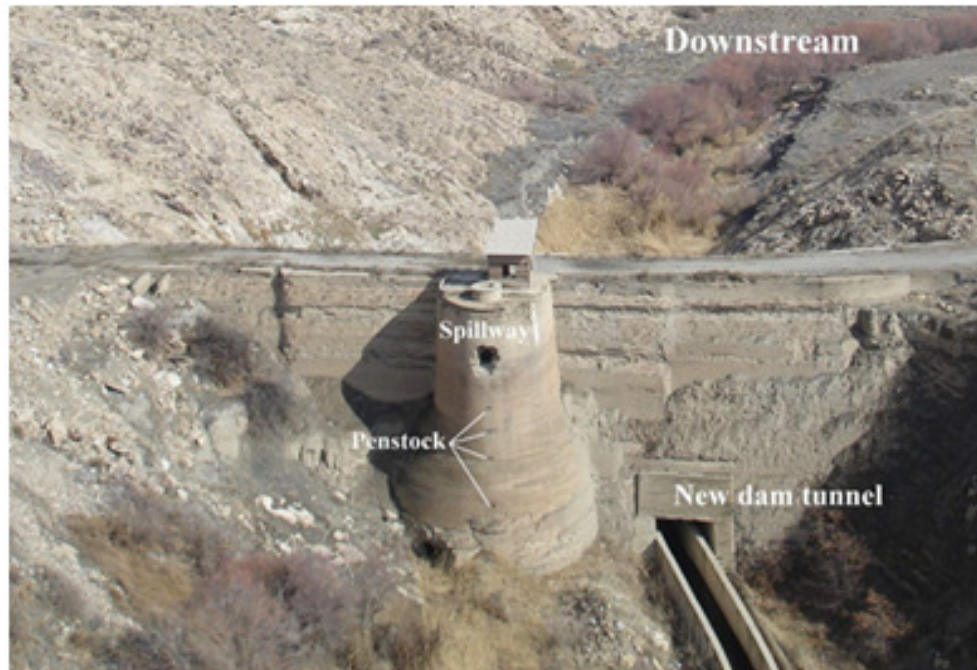
Fig. 8: Torogh dam and accessory structures
